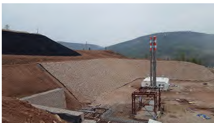
Figure 7.4.7: Technogenic surface relief within the LPG Facilities site: combination of terraces and reinforced slopes
